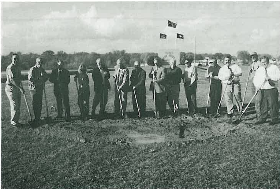
Highway Commission Chairman Herby Branscum, Jr., far right, turns the first shovel of dirt for the Highway 167 widening project.
