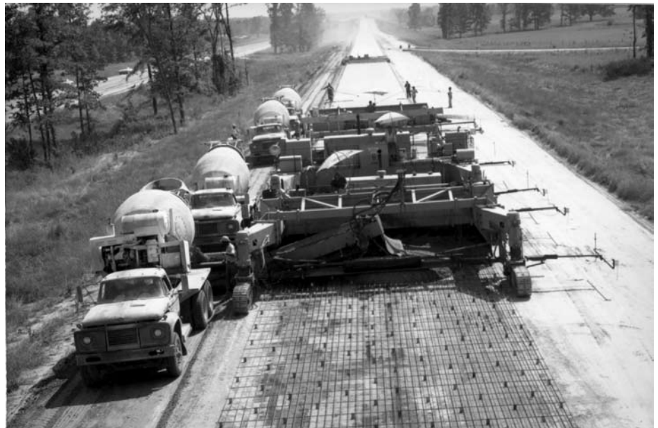
Construction on Interstate 30 near Hope in 1970.
