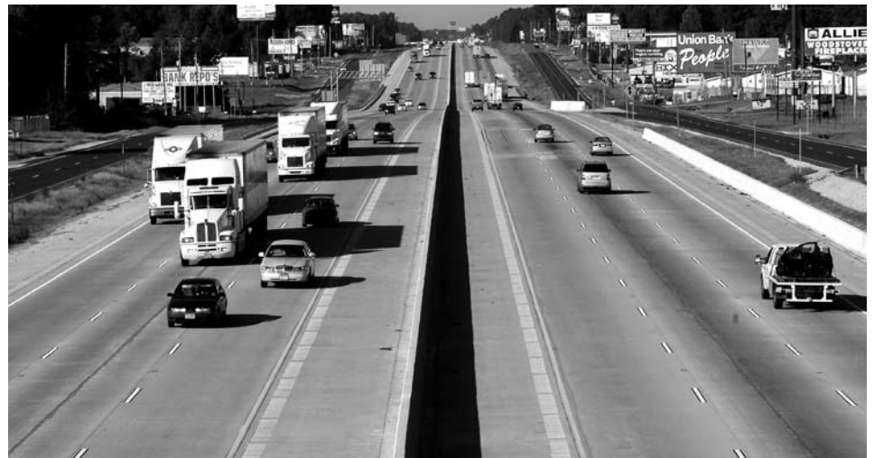
Improvements to Interstate 30 included an additional travel lane in each direction.
