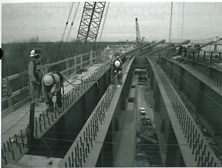
The superstructure reaches pier 36 on the Arkansas shore.
