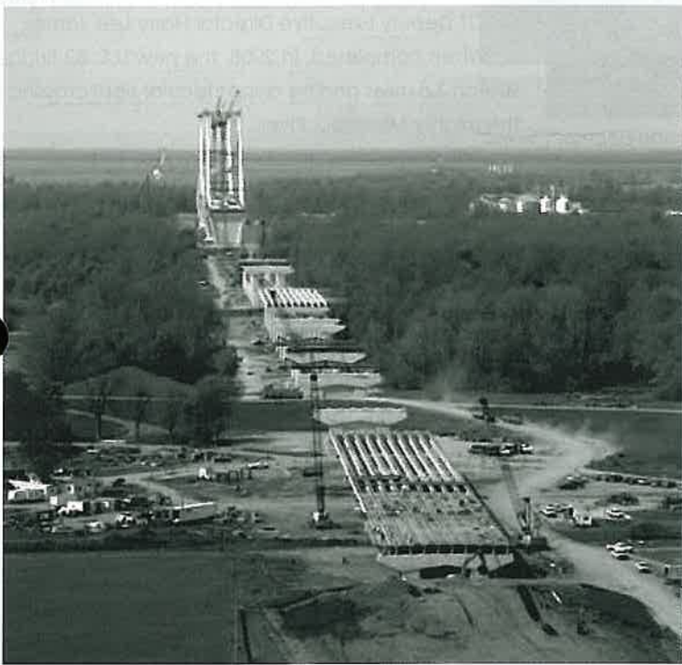
Work in progress on the Mississippi approach to the bridge.
