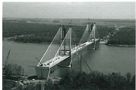
The bridge superstructure is now substantially complete.
