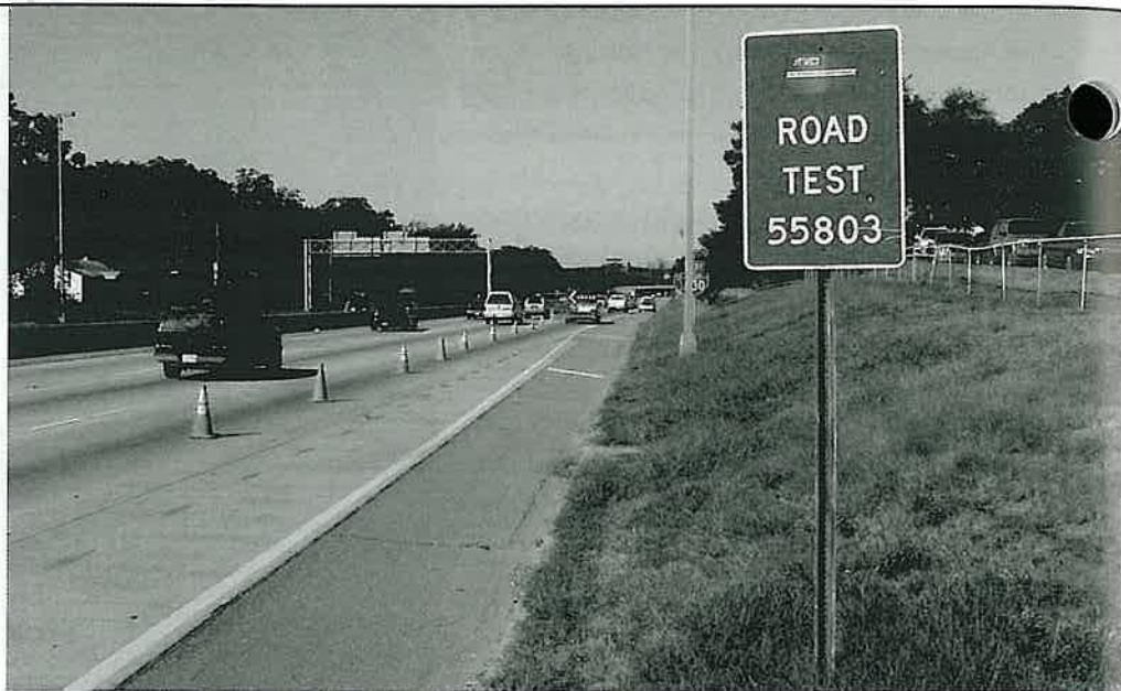
Each LTPP test section is identified with a sign such as this one on Interstate 630 in Little Rock.
