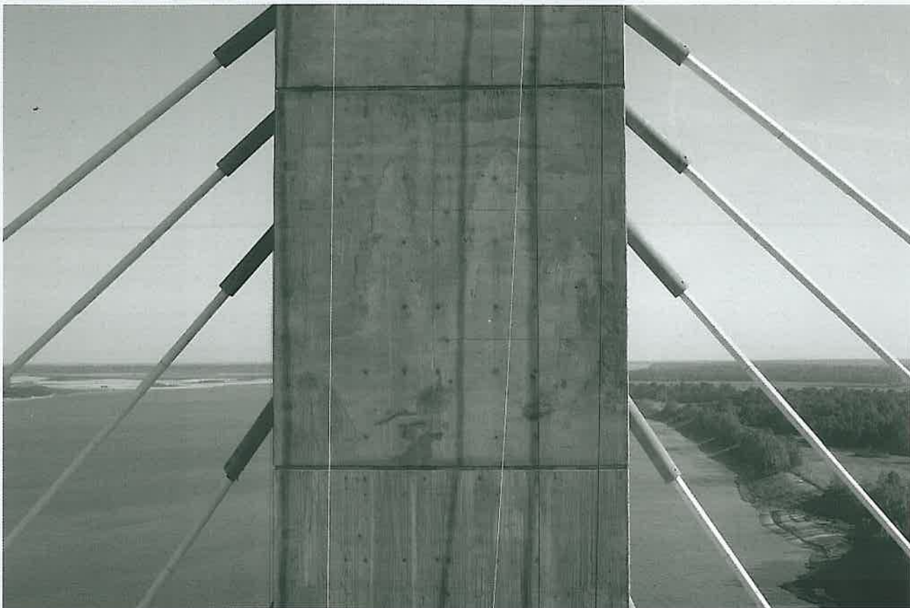
Stay cables radiate from the south tower leg of pier 37.
