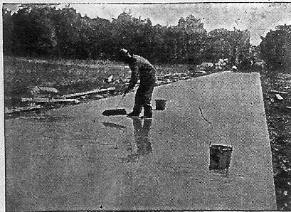
Brooming "R-B" on Road Surface
