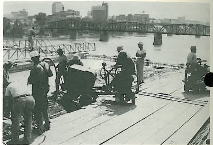
Here workmen are pouring concrete on the Freeway Bridge. The view is looking south to Little Rock.
