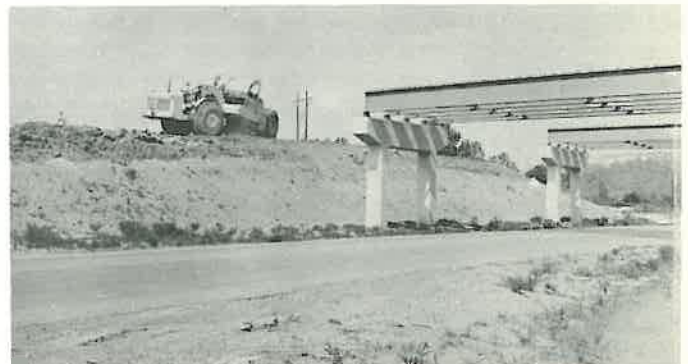
Job No. 6647. Bridges under construction over Sixty-fifth Street on Interstate 30.
