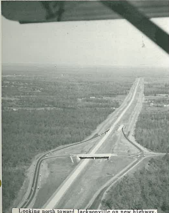
Looking north toward Jacksonville on new highway.
