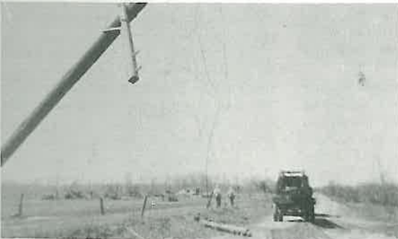
Damaged power lines, such as these, were typical all over the devastated area.
