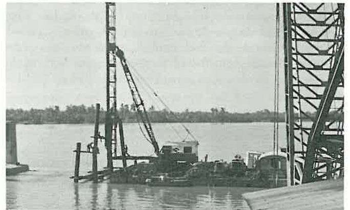
A barge is driving falsework on the Saigon River.
