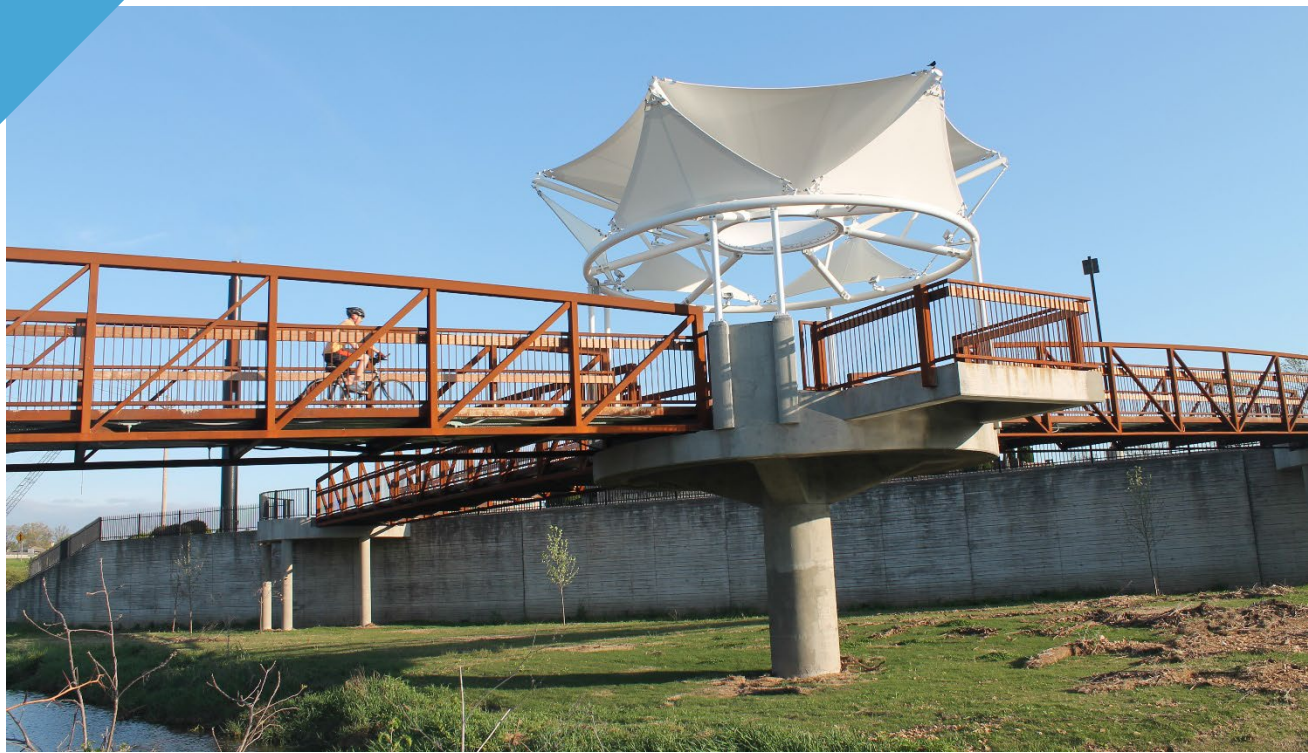
New Hope Trail Bridge, Razorback Regional Greenway, Rogers, Arkansas
