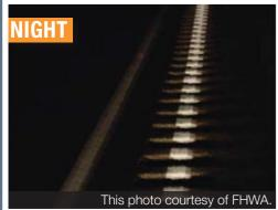
Note the brightness of the rumble strip at night, as compared to the normal pavement marking to the left of the rumble line.
