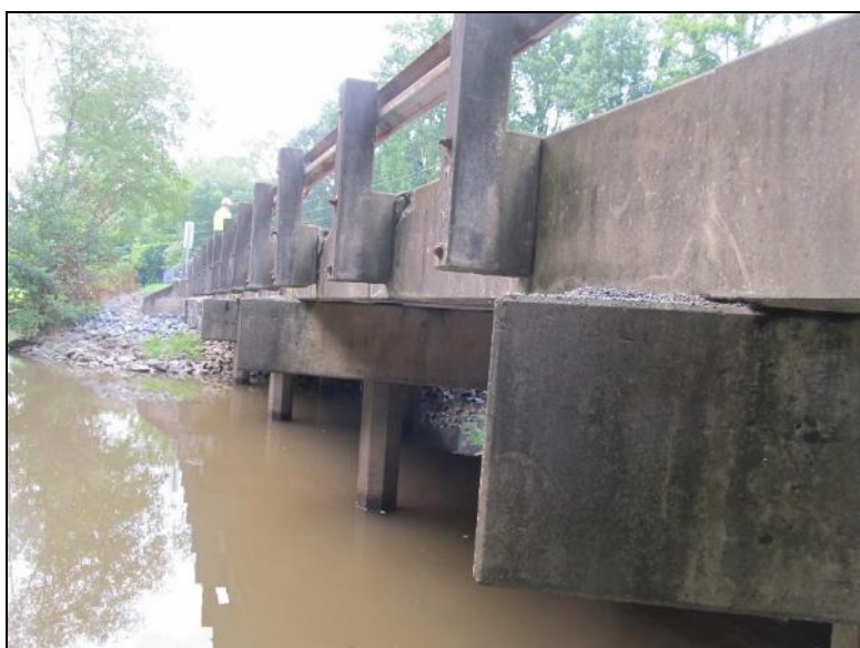
Figure 1. Bridge #03170. Reinforced concrete (RC) channel beam supported by RC pile bents with RC caps. Maximum water depth approximately 7 ft. on 7/20/2021.
