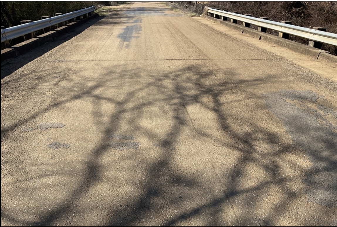
Typical deck photo asphalt overlay
