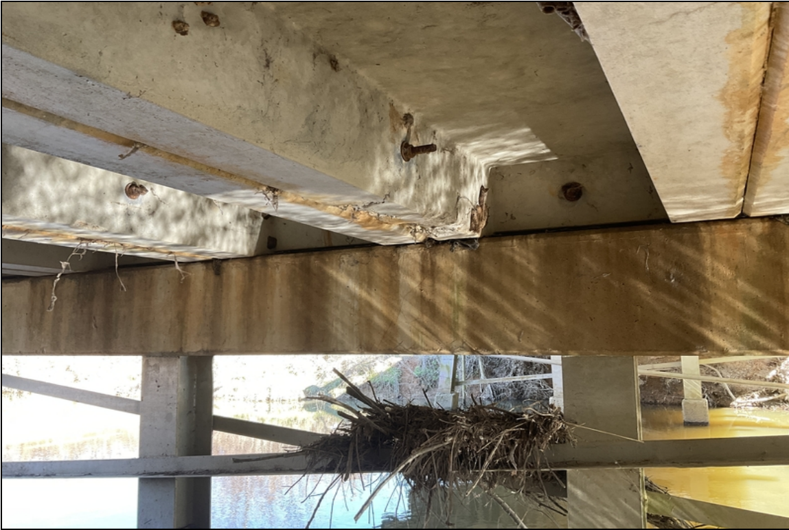
2/2022 span 3 bottom of precast unit number 3 concrete has spalled on the bottom of unit at bent 3 about 3ft long
