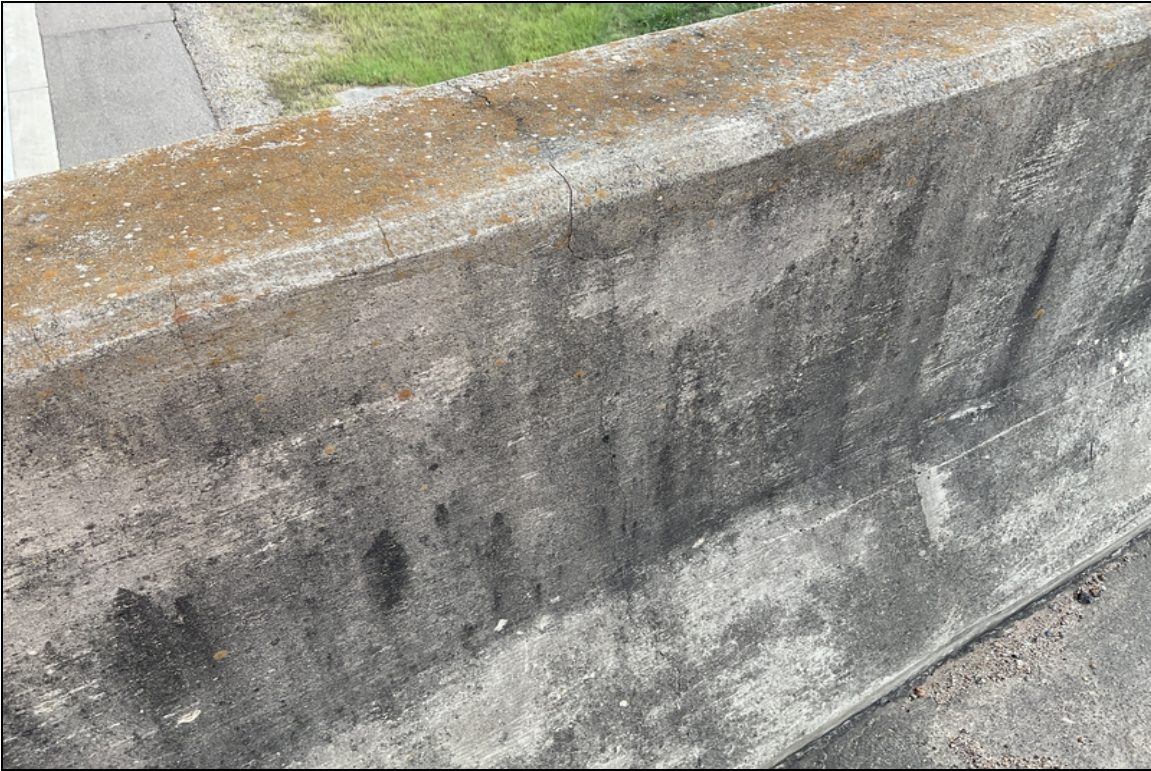
Typical cracking in the parapet wall
