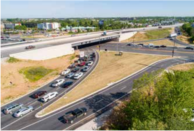
Interstate 49 and Highway 71B interchange improvements
