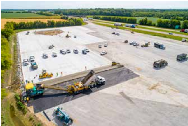
Commercial Motor Vehicle Parking on Interstate 40 in West Memphis
