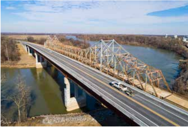
White River Bridge in Newport
