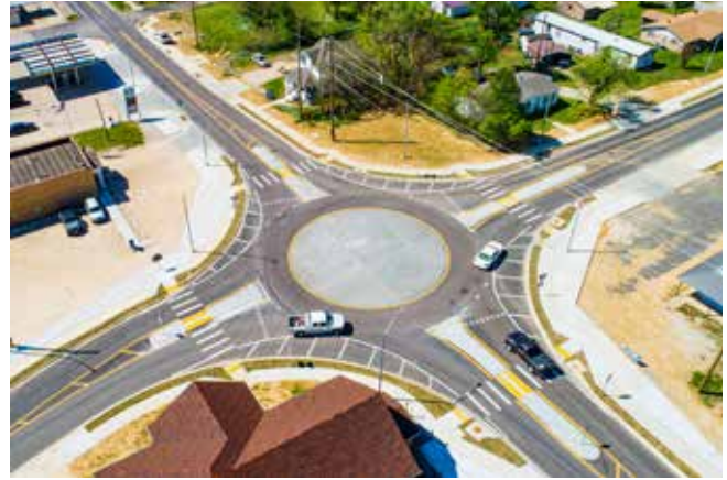
Roundabout at Highways 49 and 34 in Marmaduke
