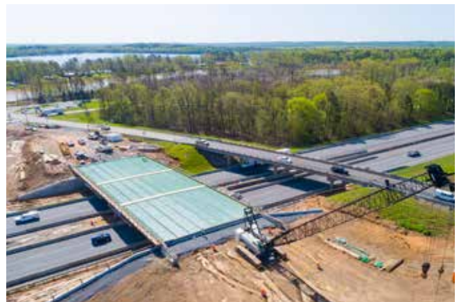
A new Highway 89 overpass over Interstate 40 at Mayflower
