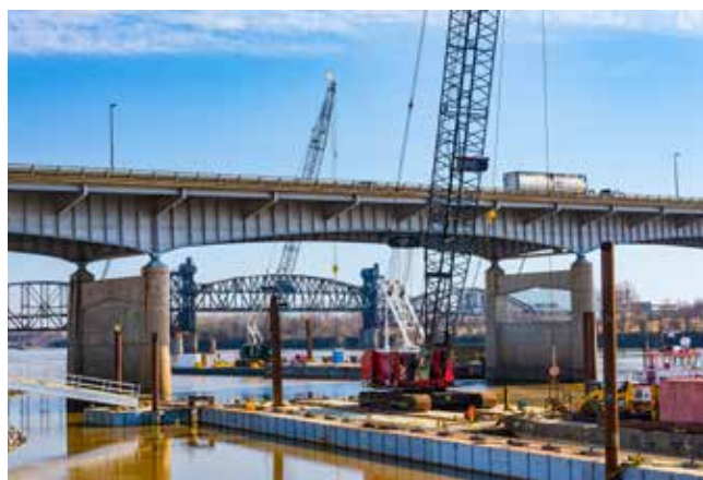
Work underway on the Interstate 30 Bridge
