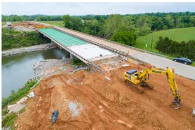
Strawberry River Bridge, Highway 56
