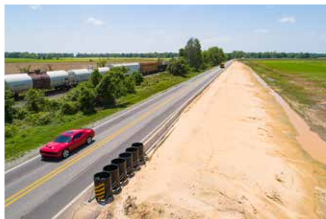
Construction on a Highway 79 passing lane
