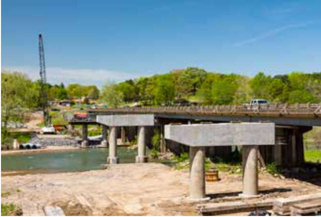
Highway 70 Glenwood Bridge over the Caddo River
