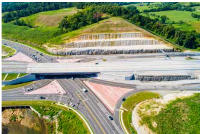
Improvements at the Interstate 49 and Highway 71B interchange
