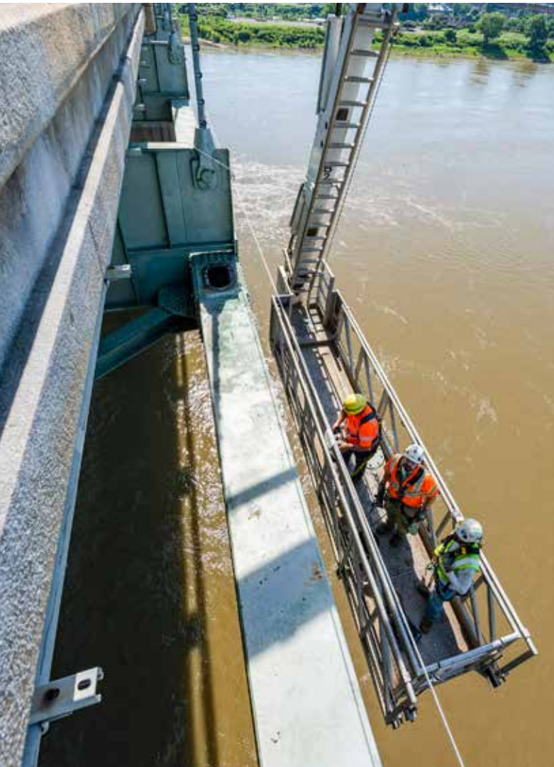
Inspecting the Interstate 40 Hernando DeSoto Bridge
