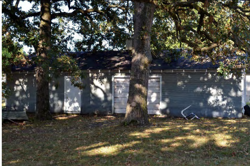
Property 21c: Southeast elevation, facing west
