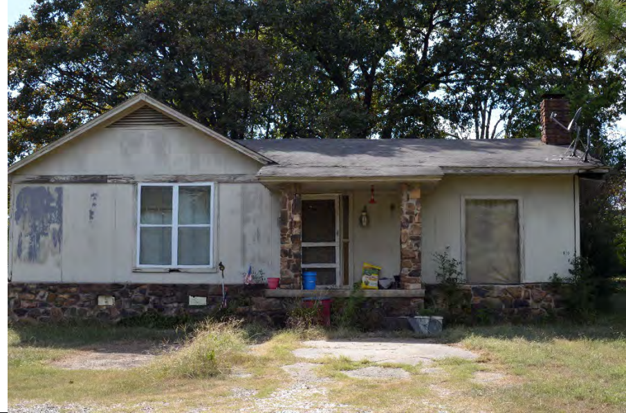
Property 17: East elevation, facing west
