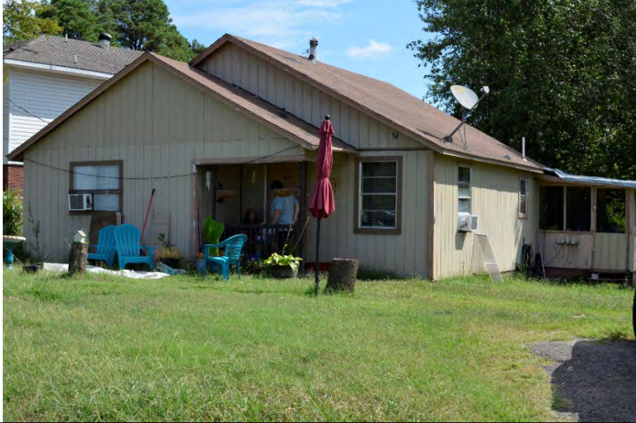
Property 7: Southwest elevation oblique
