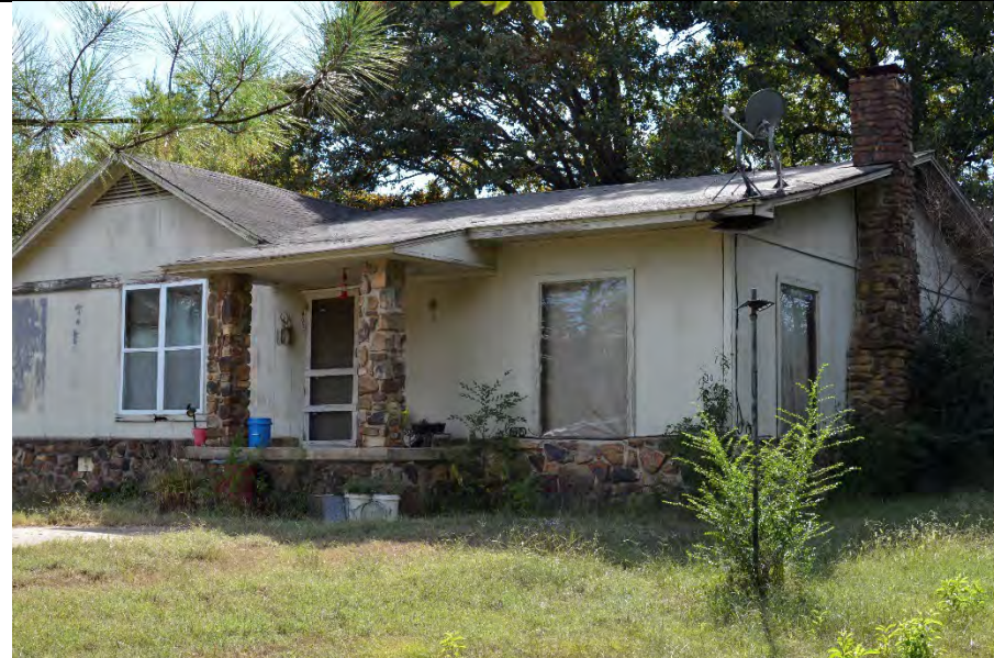
Property 17: East elevation oblique, facing southwest
