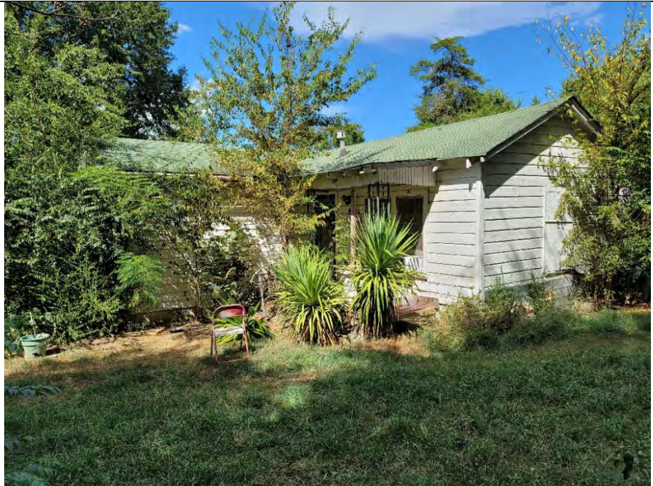
Property 13: West elevation oblique, facing northeast
