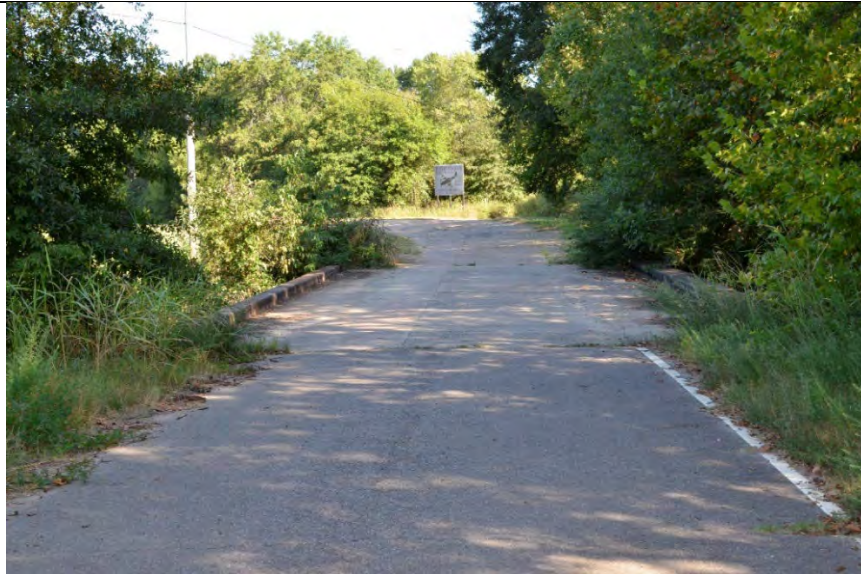
Property 23a: West Approach
