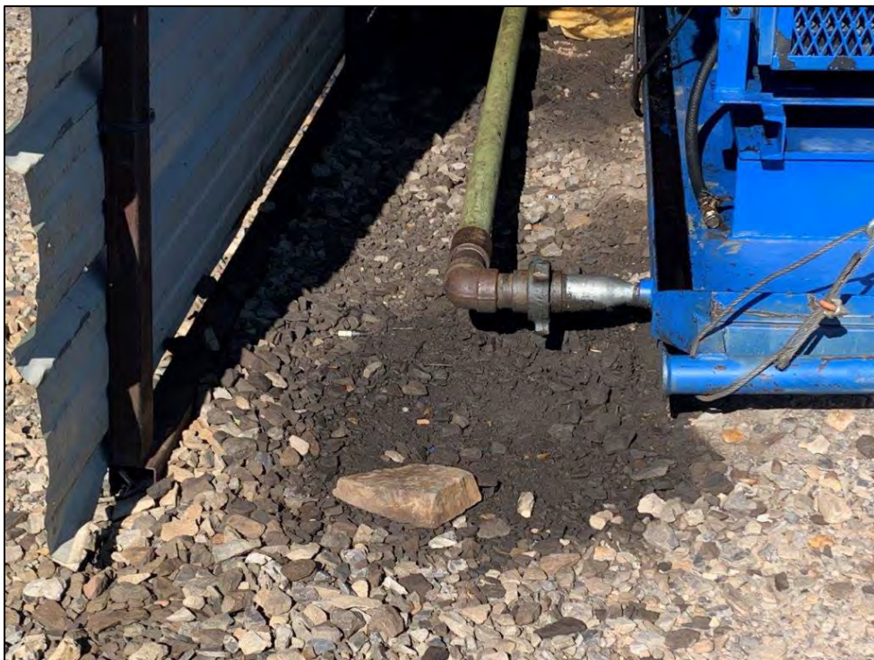
Photo 10: Close-up of oil staining on gravel at Stephens Production – Newton, Don #1 well head.
