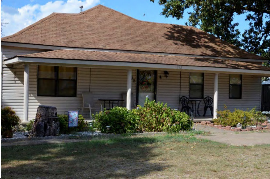
Property 15: South elevation, facing northeast
