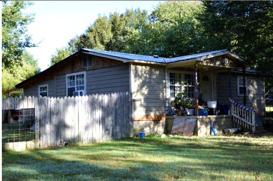
Property 18: East elevation oblique, facing northwest
