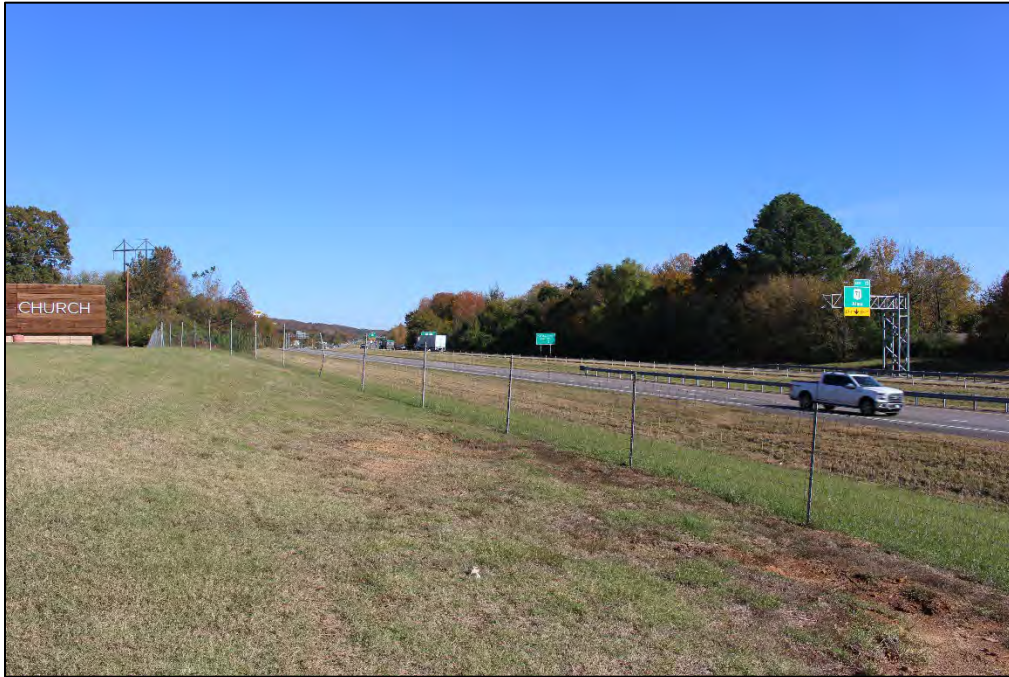
Photo 15: Looking east along I-40 (LT-2 and Validation) from 330 Rudy Rd.
