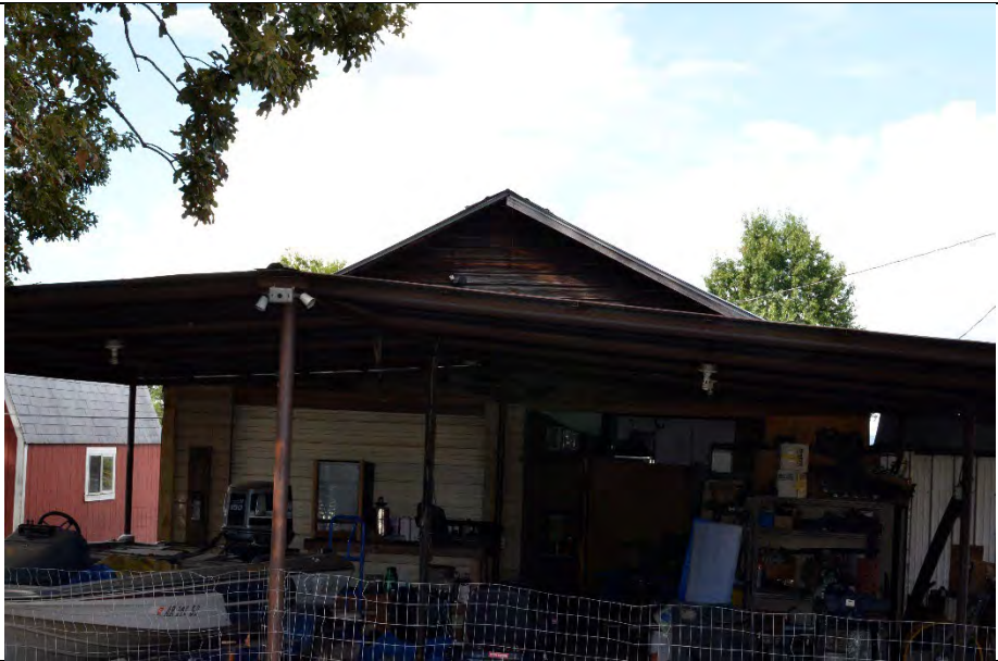
Property 15a: South elevation detail, facing north
