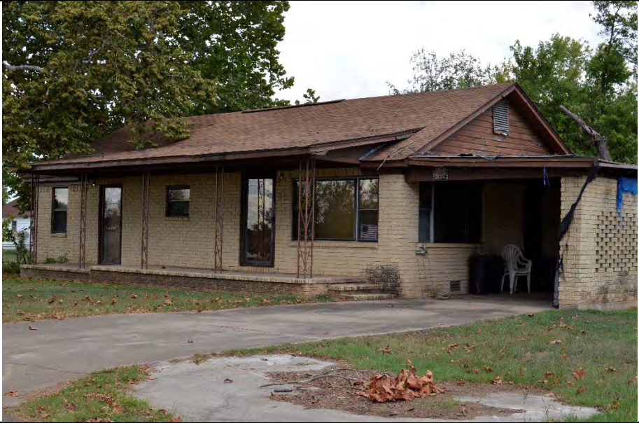
Property 1: 1024 Church Street (1r), facing northwest
