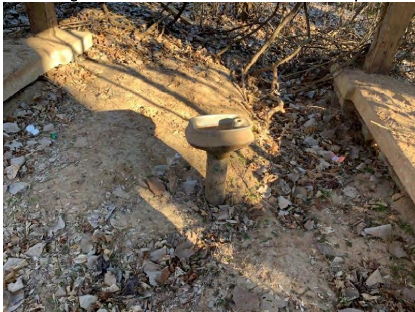
Figure 5-6: Abandoned Water Fountain Close Up
