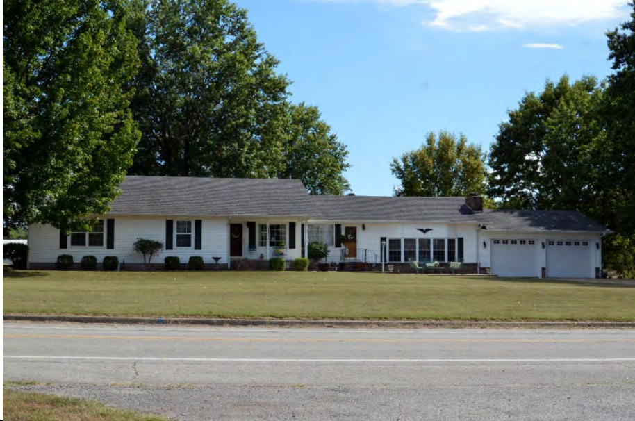
Property 16: North elevation, facing south
