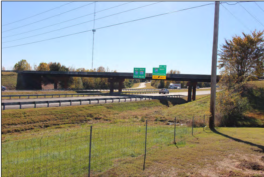
Photo 16: Looking west along I-40 (LT-2 and Validation) from 330 Rudy Rd.
