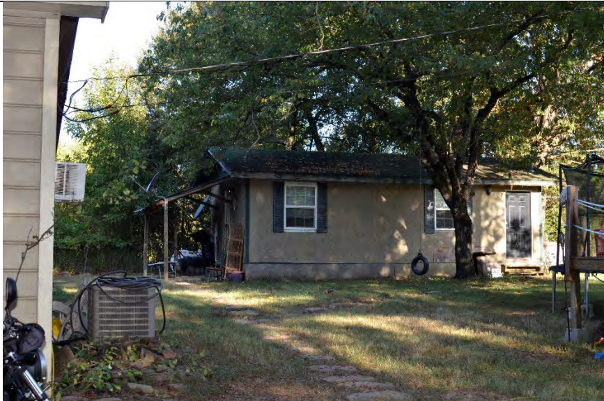
Property 18a: East elevation, facing west
