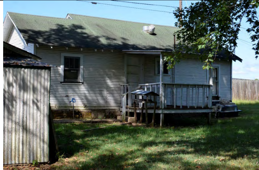
Property 9: Rear (northeast) elevation
