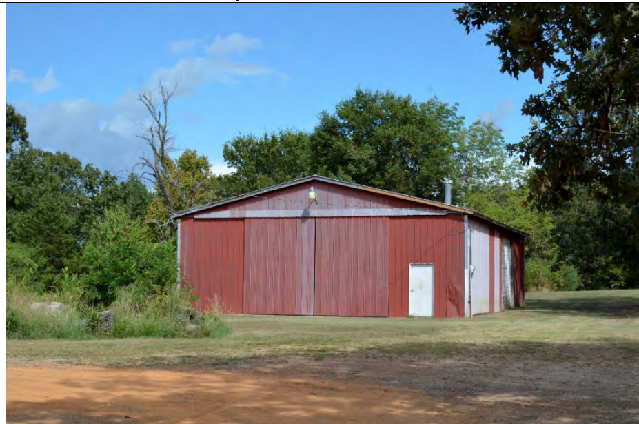
Property 11b: West elevation, facing east
