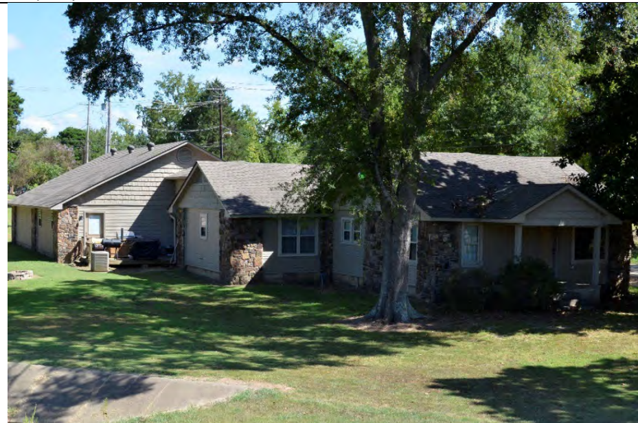
Property 10: Oblique featuring the south and west elevations
