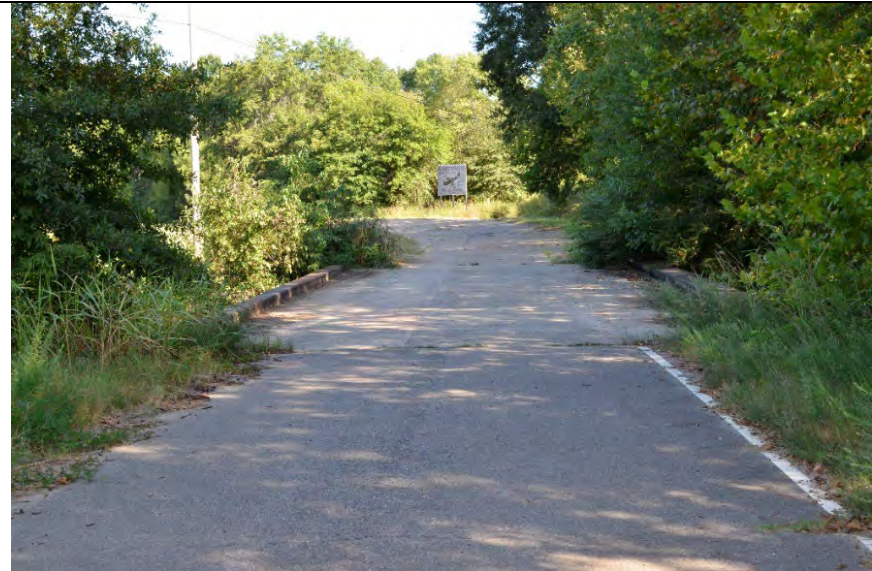
Property 23: Slab bridge (Property 23a), facing northwest
