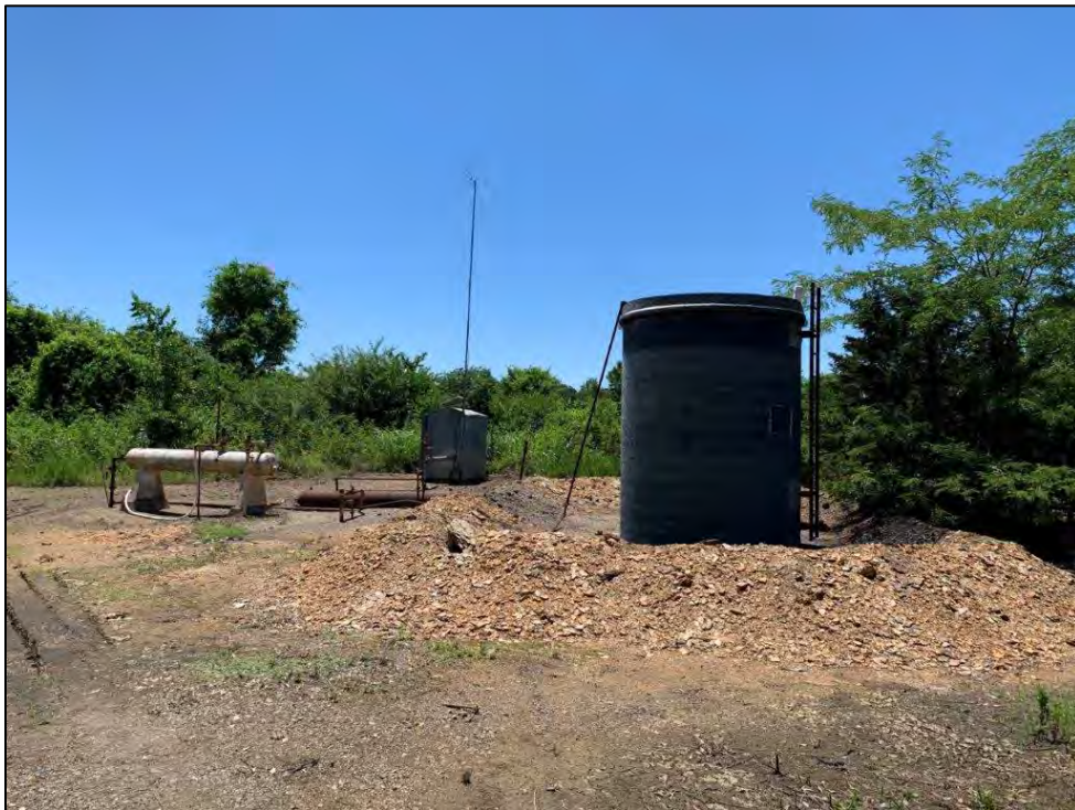
Photo 2: View southwest of Brown 1-1 well pad (Exhibit 2, Map ID #3) with produced water tank and gas/water separator.
