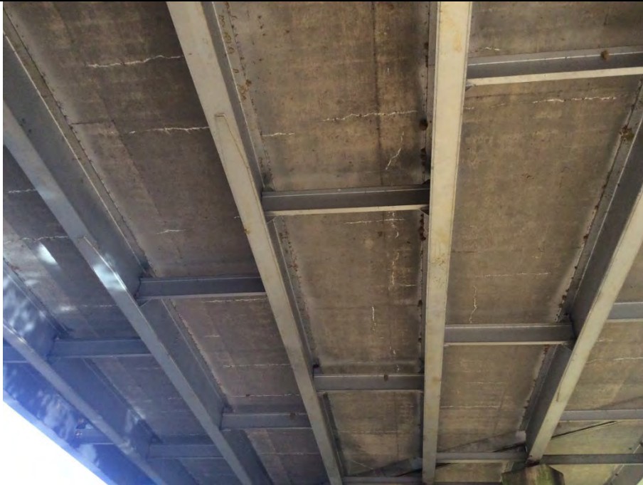
Property 4: Bridge substructure
