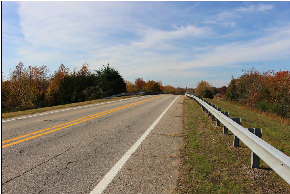
Photo 12: Looking west along (ST-5) Collum Ln. towards bridge over I-49.
