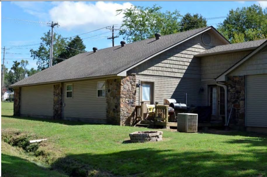
Property 10: West elevation, non-historic gable addition
