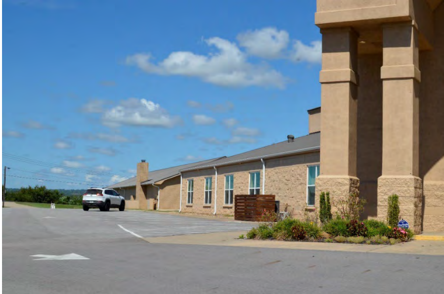
Property 2: South elevation, c.1972 front-gable building and c.2001 addition
