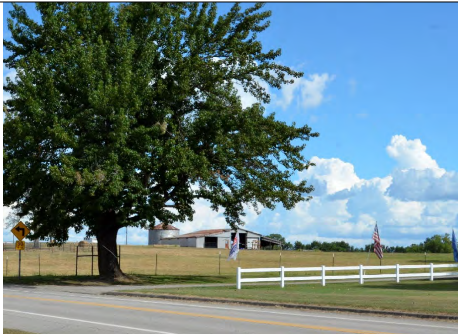
Property 14: West elevation, facing southeast
