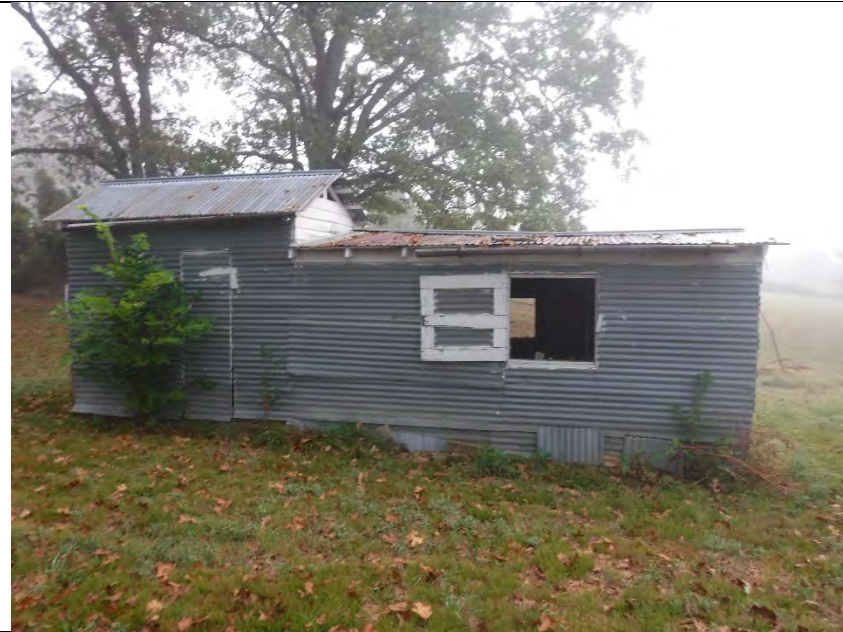
Property 21b: East elevation, facing west
