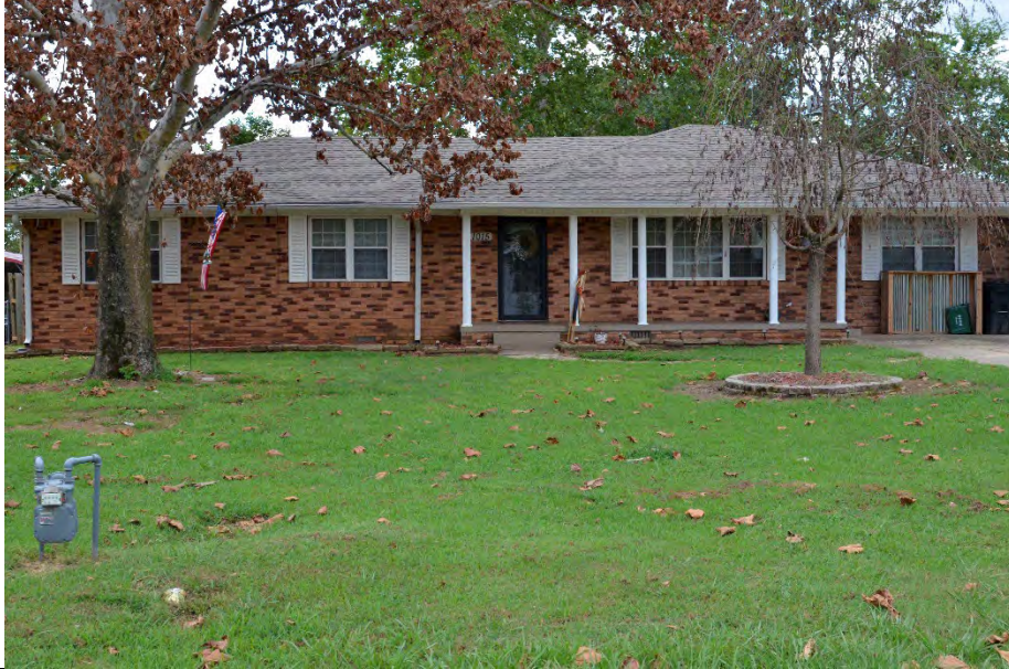
Property 1: 1015 Church Street (1o), facing south
