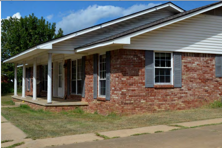
Property 11: West elevation oblique, facing northeast
