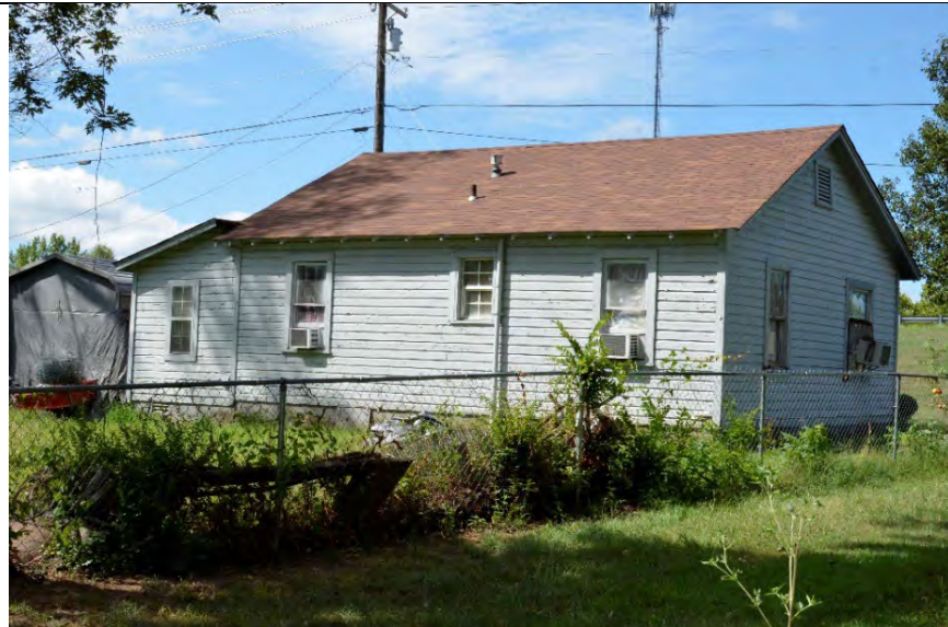
Property 8: Rear (northeast) elevation
