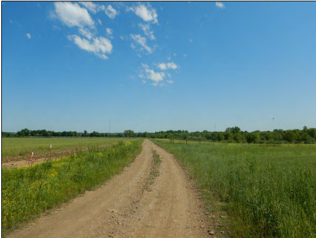
Figure 4-6: Middle Portion of Road Segment, Camera Facing North
