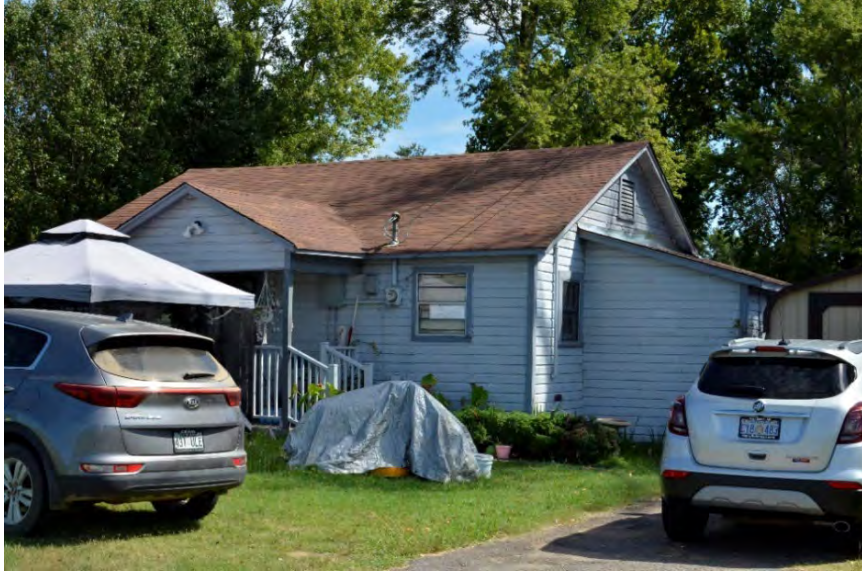
Property 8: Front (southwest) elevation
