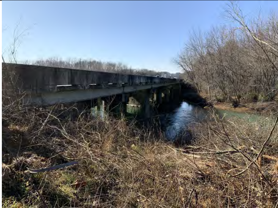
Property 3: Bridge substructure
