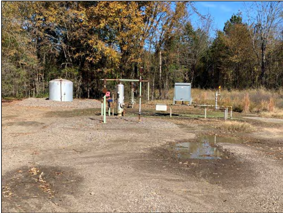
Photo 5: View north of Stephens Production – Steward Gillie Smith #1 well head ( Exhibit 1, Map ID #3; Exhibit 2, Map ID #1 ) located north of Clear Creek Road 0.5-mile east of the intersection with Highway 162 in Kibler. This was the only site identified on both the regulatory and natural gas well database searches.
