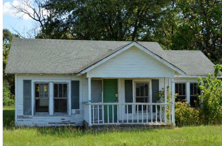
Property 9: Primary (southwest) elevation
