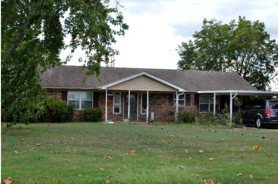
Property 1: 1023 Church Street (1q), facing south
