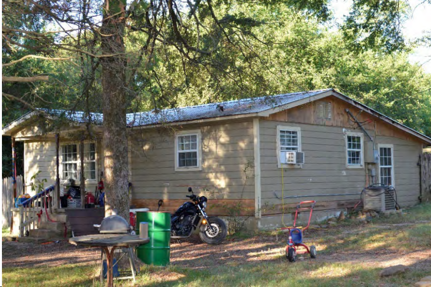
Property 18: East elevation oblique, facing southwest
