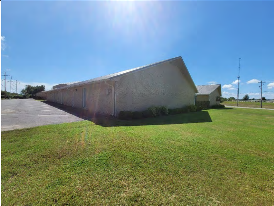
Property 2: North elevation oblique, c.1972 front-gable building
