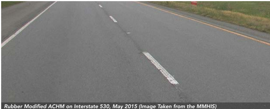
Rubber Modified ACHM on Interstate 530, May 2015 (Image Taken from the MMHIS)
