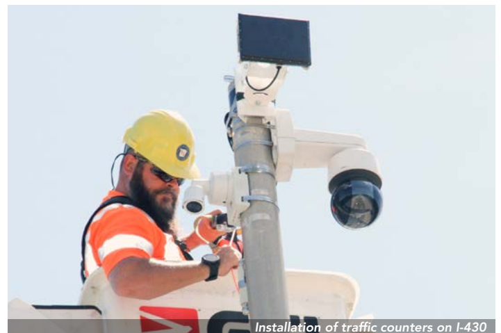
Installation of traffic counters on I-430
